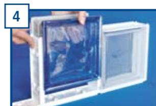
**UK** Place the glass blocks in between the vertical profiles until the row is completed (photo 4).
