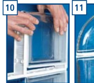
**UK** Finish the joints with quick-setting mortar.
