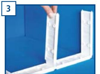
**UK** Once all the horizontal profiles have been positioned, start inserting the vertical profiles by inserting them into the slits according to the glass block chosen (Pegasus or Basic). (Photo 3).
