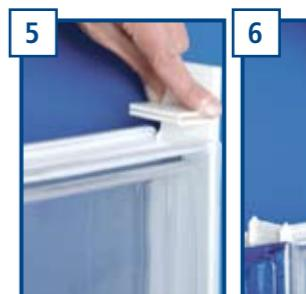
**UK** Insert a "T" shape cross into the top block leaning against the wall (laterally) in order to continue the installation process with VetroCLICK (photos 5, 6, and 7).
