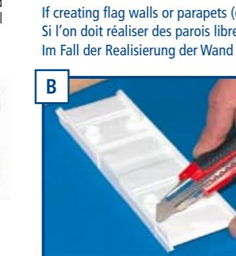
**UK** Cut the profile in correspondence of the score line that marks the end block of the wall or rectangular block (photo B, point 1).
