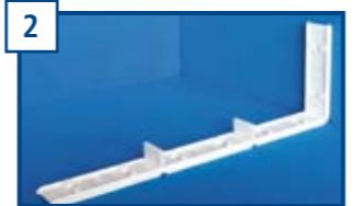
**UK** Cut a cross into a "T" shape (photo A) and join it to the profiles. Continue to add profiles and crosses, repeating the drawing, drilling and screwing operations until reaching the desired width of the wall (photo 2).
